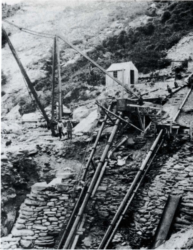
The hydraulic elevator at Choie Sew Hoy's gold mine at Nokomai, Otago. Sew Hoy was one of the leading gold-mining businessmen in the province. (Hocken Library)
