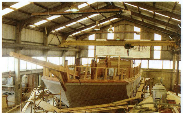
The Freightways scow, TED ASHBY, under construction.
